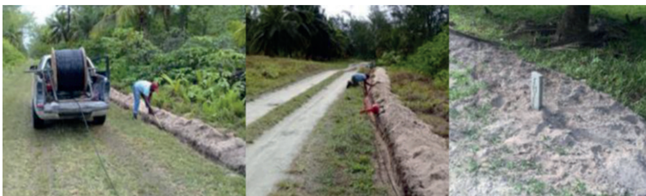
Laying of inland fibre in North and South Islands of Agalega
